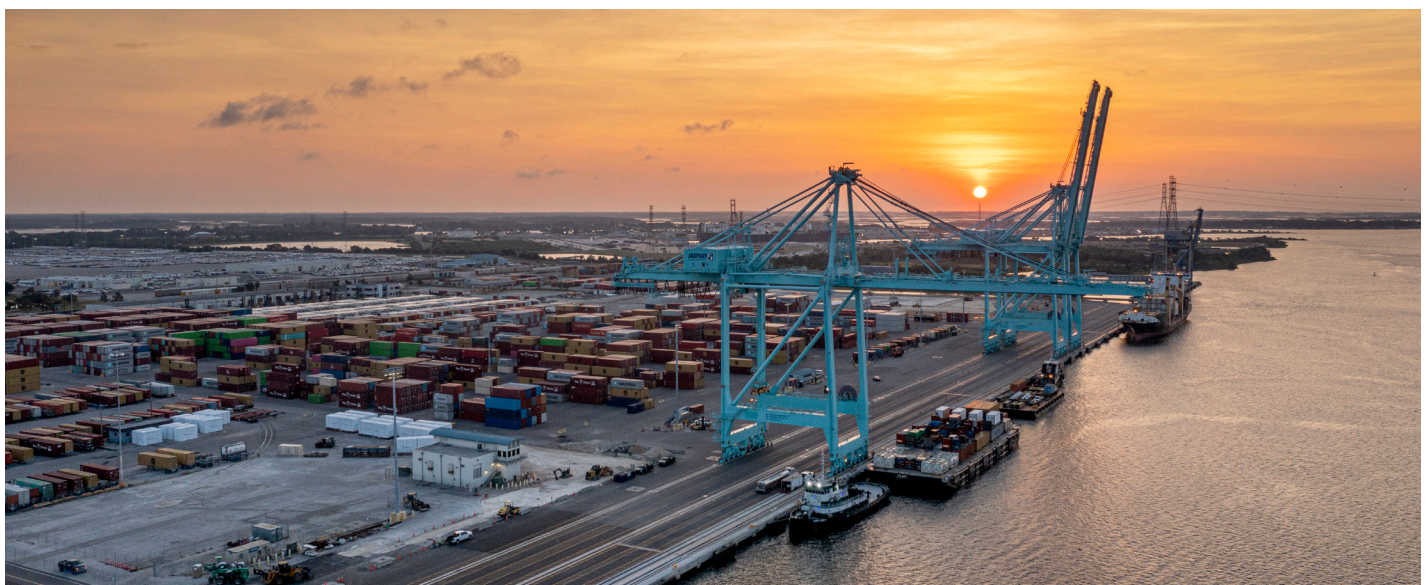
Bulkhead seawall at the Port of Jacksonville in Florida.
