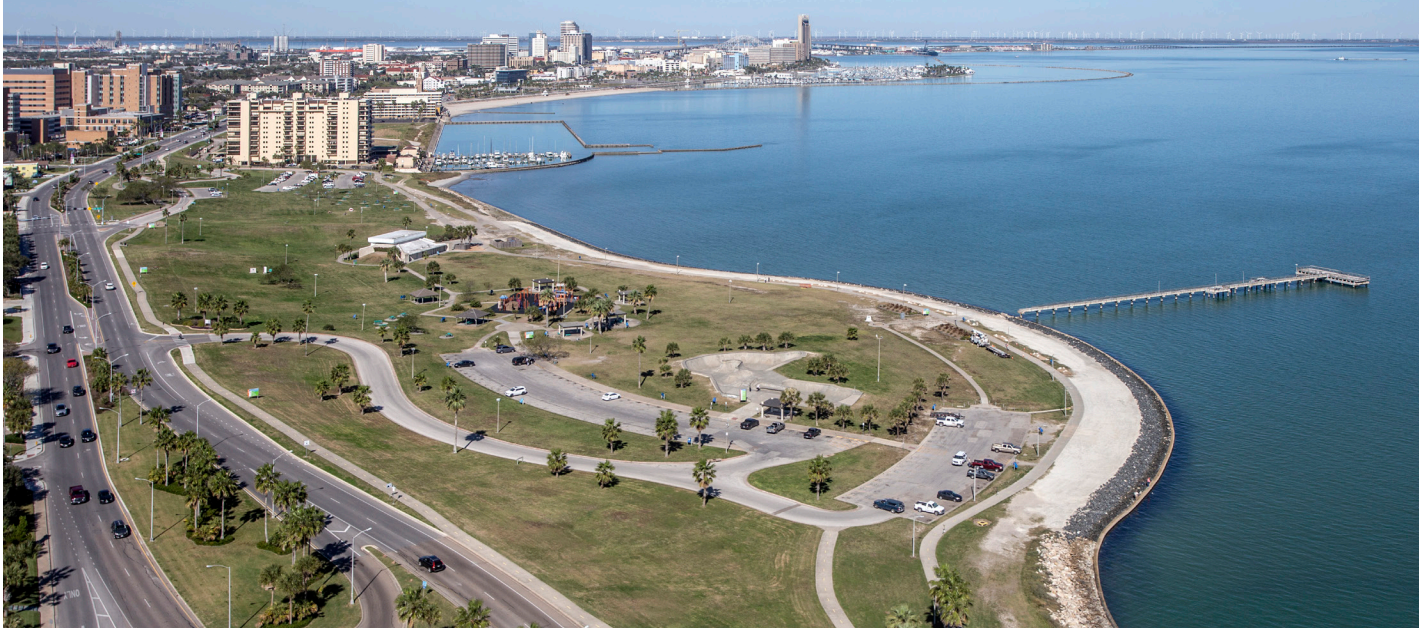
The seawall at Cole Park in Corpus Christi, Texas.
